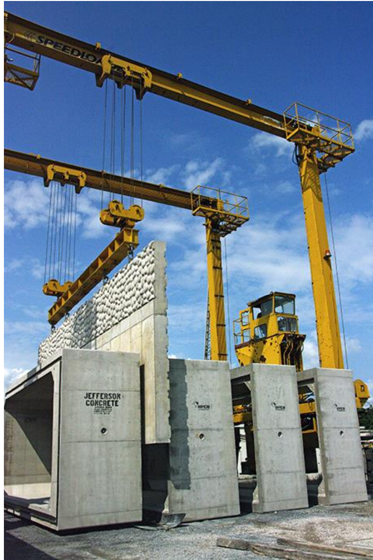
Figure 1.7: Prefabricated Girders being lifted with two cranes at bridge (NPCA)
