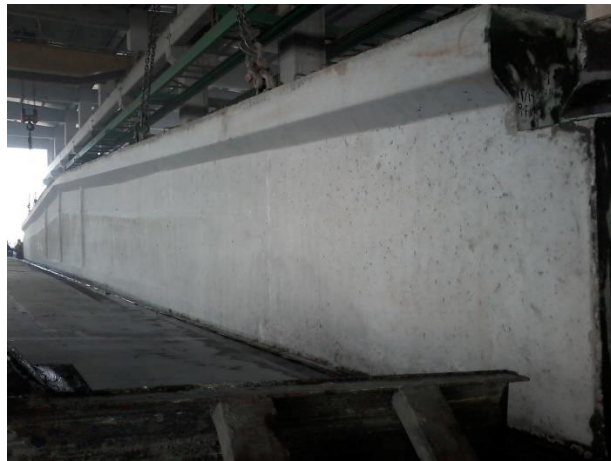
Figure 3.7: Rafter beam being cured
