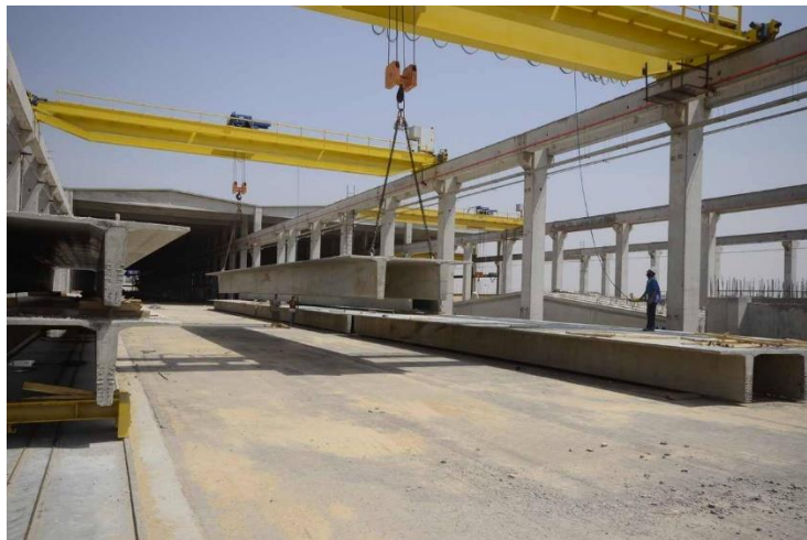
Figure 3.5: Image shared by contractor showing Fixed crane moving Double T Slab
