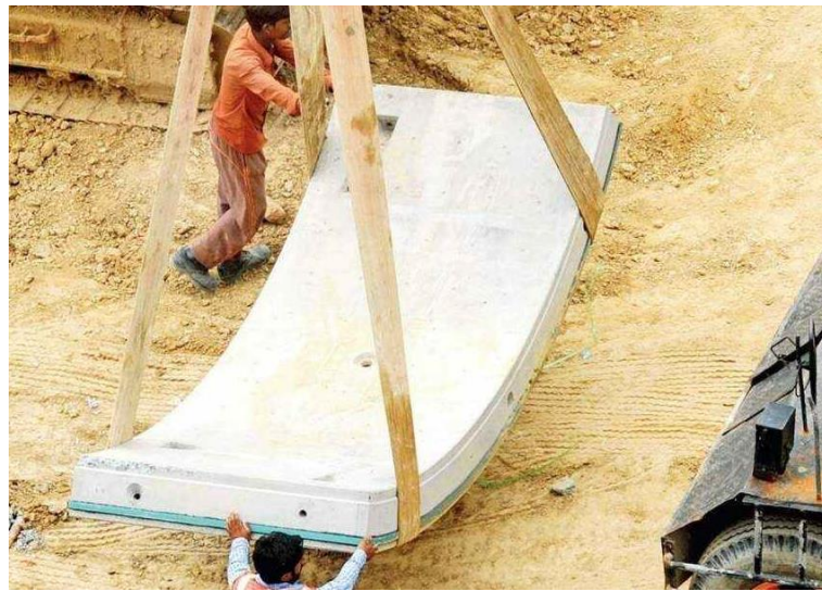
Figure 1.5: Crane lifting precast panel mold (Hegart et al., 2020)
