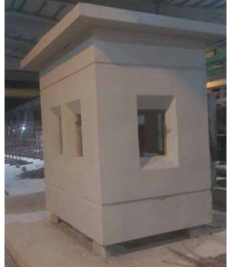
Figure 3.4: Precast Guard Room curing after production
